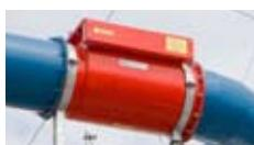
*In order to safeguard an EX installation an isolation valve prevents explosions from going back into the system*
